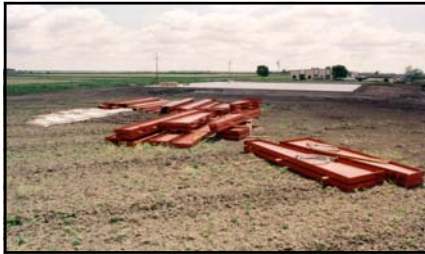
A conventional metal building is delivered in pieces (purlin/girt structure with loose sheeting and insulation).
