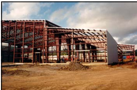
Field framing of window and door openings are required. Loose sheeting is field-attached to wall girts and roof purlins.
