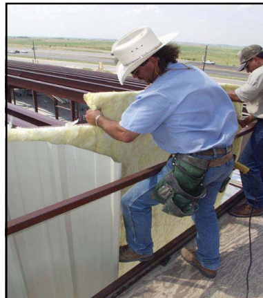
Field framing of window and door openings are required. Loose sheeting is field-attached to wall girts and roof purlins.
