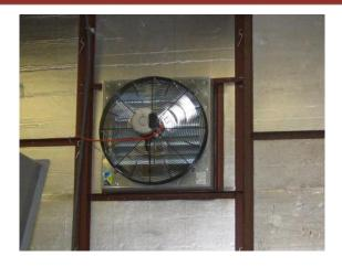
Wall Panel with Factory Installed Louver and Exhuast Fan
