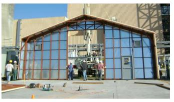
Endwall Being Set with Factory Installed Personnel Door,
