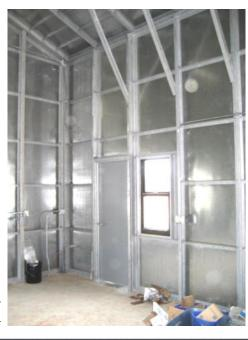
A Building's Interior with Hot-Dip Galvanized
