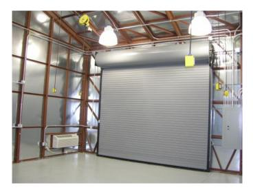
Galvanized Steel Liner Galvanized steel liner with red primer panel frames.
